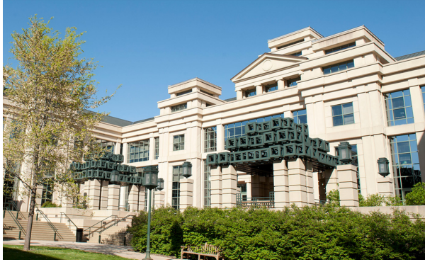
Figure 1: Pappajohn Business Building
