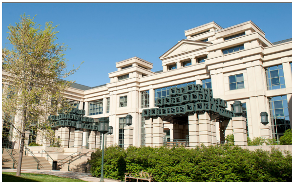
Figure 1: Pappajohn Business Building
